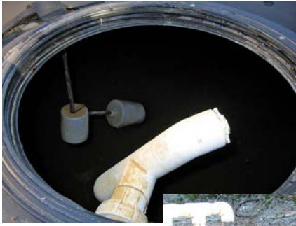
A float switch in the secondary tank controls the pump that draws from the primary tank.
