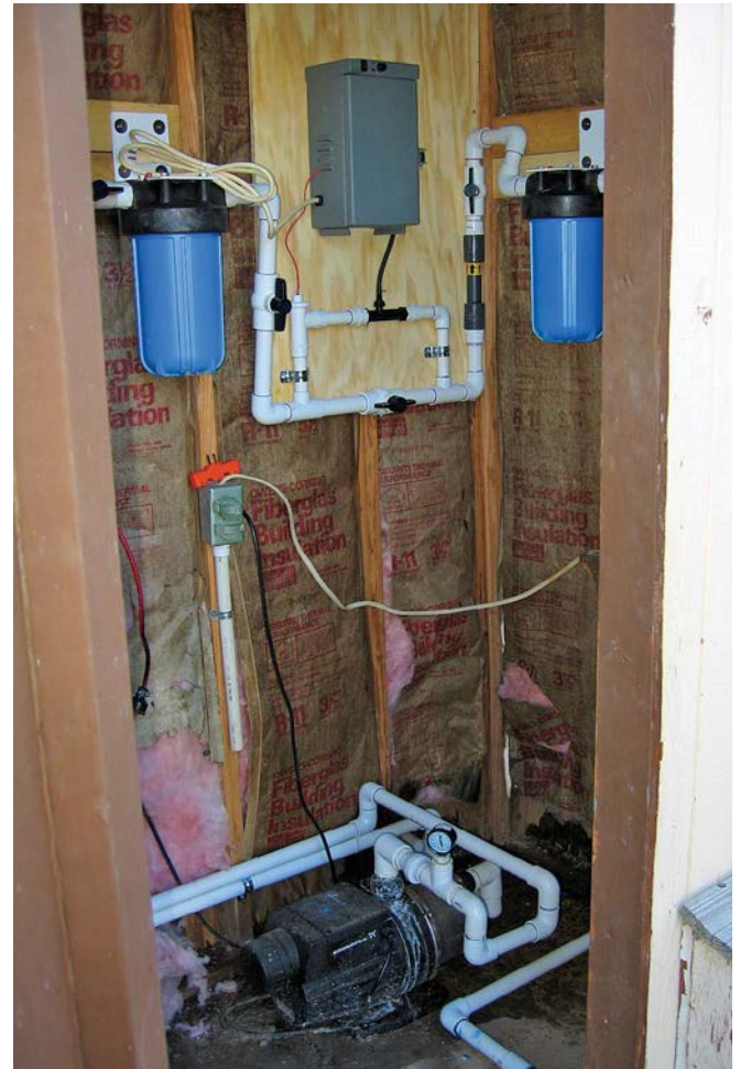
A Grundfos pressure-booster pump (bottom) provides the house’s water pressure through a two-stage filter and ozone purification system (top).
