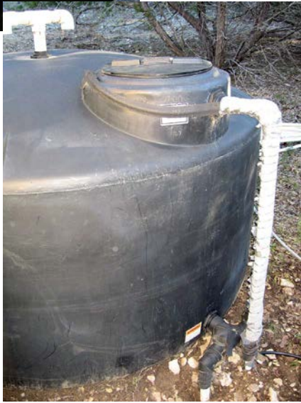
The 1,200-gallon secondary tank served as the original water storage. Now, it provides additional capacity and a place for incoming water to cool in the shade before entering the house.
