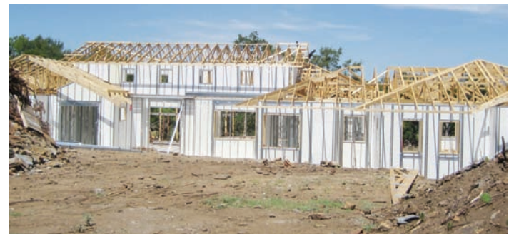
The Wilkens home is framed with foam and steel panels with metal studs. There is no wood in the lower part of the house and the insulation is 5 1/2" foam. “We are basically living in a large cooler,” said Karen.
