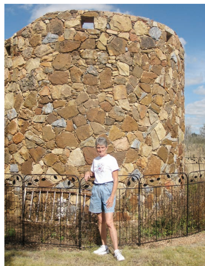
Karen Wilkins is pictured in front of the 10,000 gallon cistern she and her husband Joe first envisioned after seeing a similar one on a trip to Italy and Greece. Inside the rock façade is a fiberglass tank surrounded by cinder blocks, mortar and rebar.
