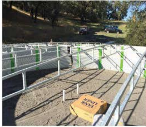
Roof truss construction.
