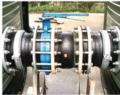
Tanks fitted for municipal water storage.
