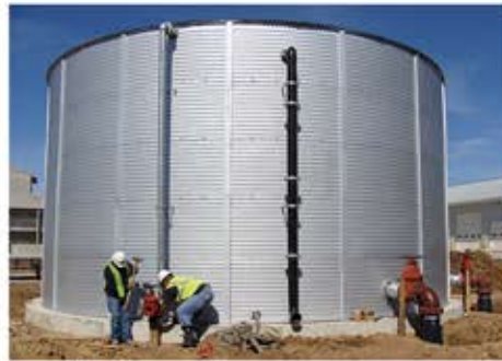
Industrial water storage tank.
