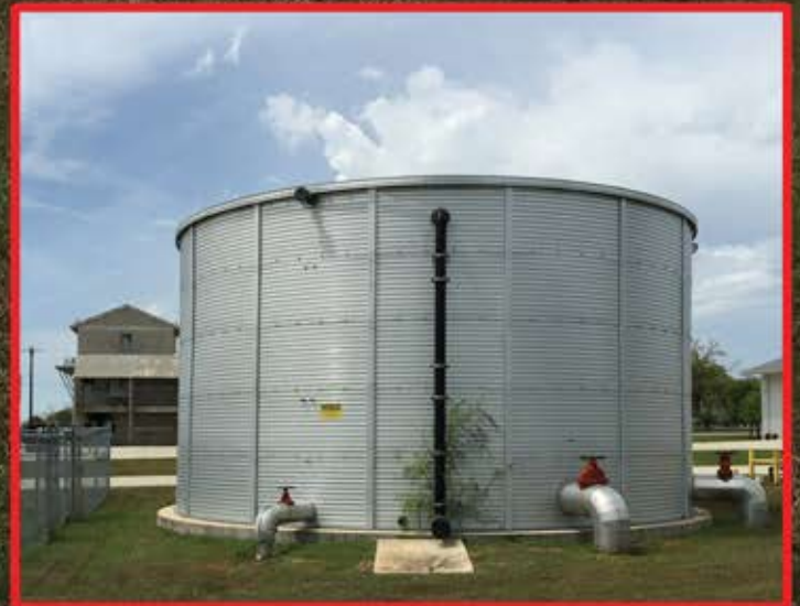
Two 100,000 gallon Pioneer fire tanks at the First Responders Academy in San Antonio, Texas
