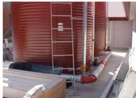
Fire water tanks.
