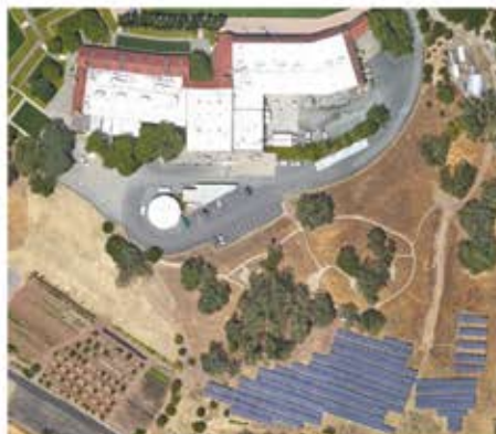
Water storage and solar panels, a truly sustainable winery.
