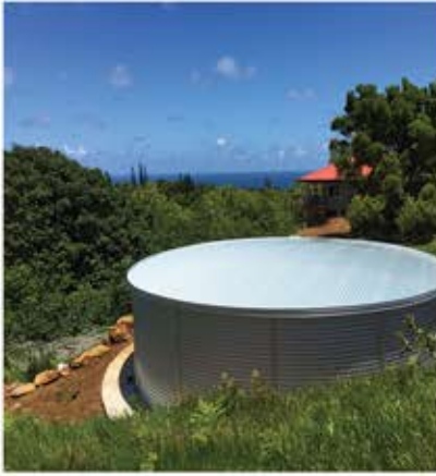
29,173 gallon tank in Hawaii.
