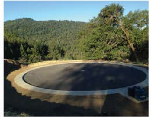
An example of a well-constructed ring beam foundation.
