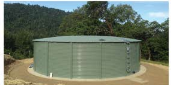
Completed tank, ready for anchoring.
