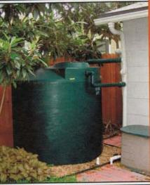
High-density polyethylene (HDPE). Used above grade or below grade, this material's capacity ranges from 50 gal. to 12,000 gal. The average price runs about \$1 per gal.
