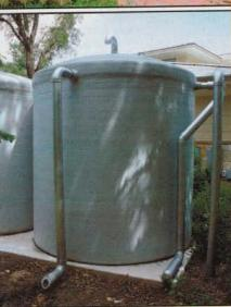
Fiberglass. This material can be used above grade or below grade. Manufacturers can make larger tanks (up to 20,000 gal.) because the material is stronger than HDPE. The average price is \$2 to \$3 per gal.
