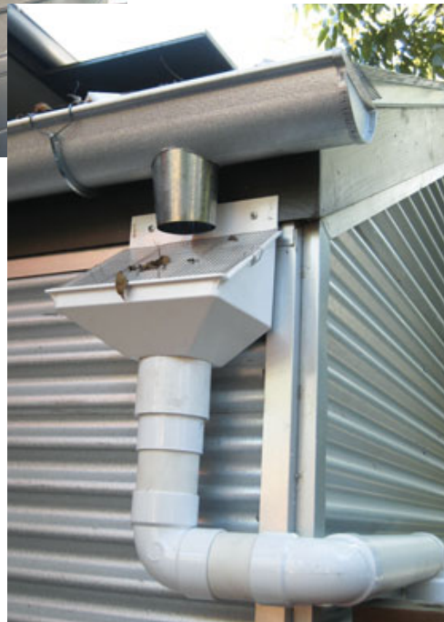
Figure 3. Solid debris such as leaves and twigs are kept out of the system by screening the tops of the gutters (above) and installing a rain head (right) in the downspout. The sloped screen of the rain head diverts debris into the yard while allowing water to pass through. A second, finer screen underneath prevents mosquitoes and other insects from getting into the tank.
