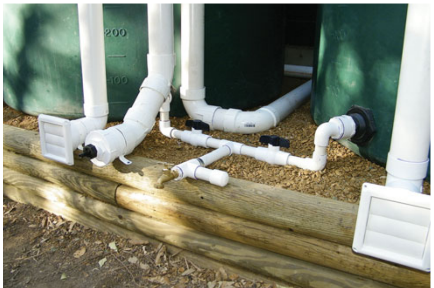
Figure 6. The overflow pipes on this nonpotable system terminate at louvered vents (designed for clothes driers), which open as the water escapes, then close to keep insects out. The black fitting to the right of the louver (above) is the dripper valve that drains the first-flush diverter. This simple system has no pump; water is drawn by gravity from the hose bib between the tanks.
