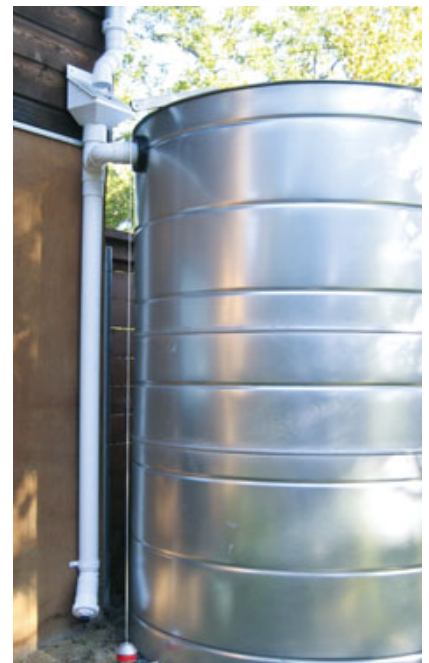
Figure 1. In a dry-pipe system, the tank is placed close to the house and the rainwater flows straight down and in through the tank inlet. Shown in the photo above is a custom steel tank with a rain head and a tall diverter pipe.
